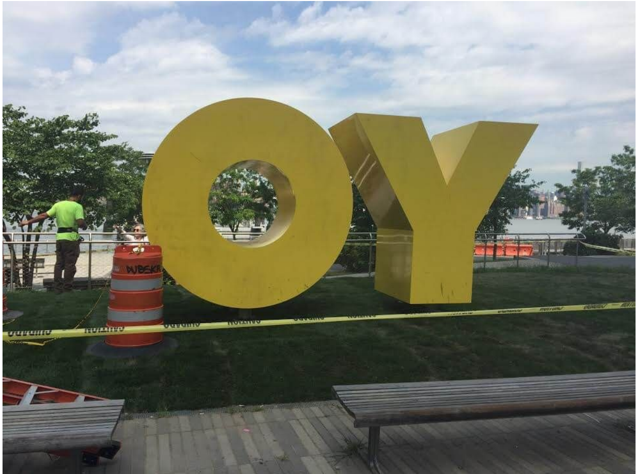
The sign being installed Monday. Photo from a Brownstoner tipster
